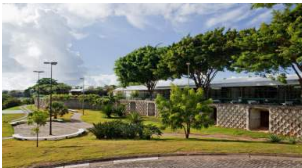
Figura 09: Vista externa do Hospital Sarah Kubitschek
