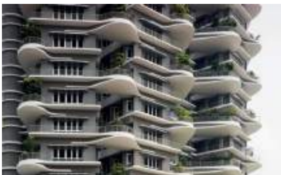
Figura 22: Vista das janelas do Hospital NG Teng Fong
