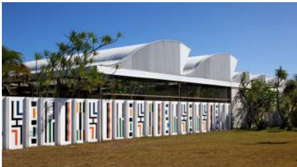
Figura 11: Vista dos Sheds na fachada Hospital Sarah Kubitschek
