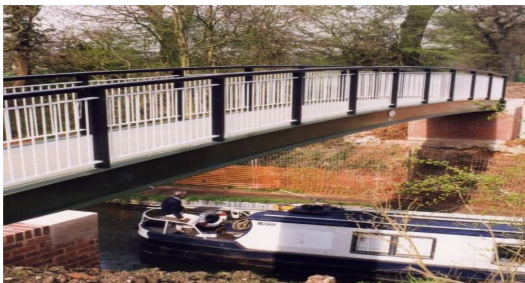
Figura 10 - Passarela Redrow Footbridge, West Midlands/UK
