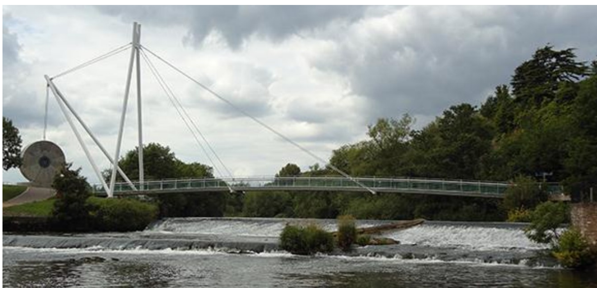
Figura 15 – Miler's Crossing Bridge, Exeter/UK
